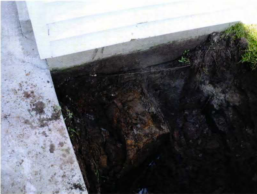
Picture 3: UST 260Beech-2 excavation.
