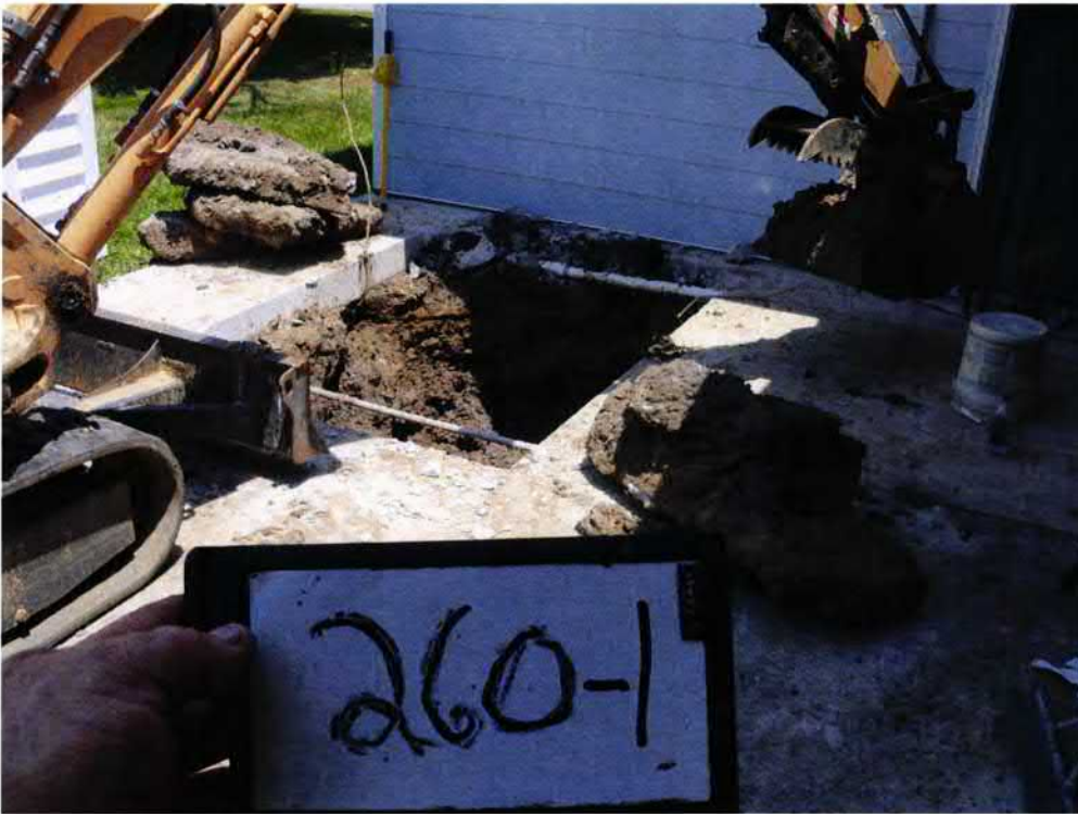
Picture 2: UST 260Beech-1 excavation.
